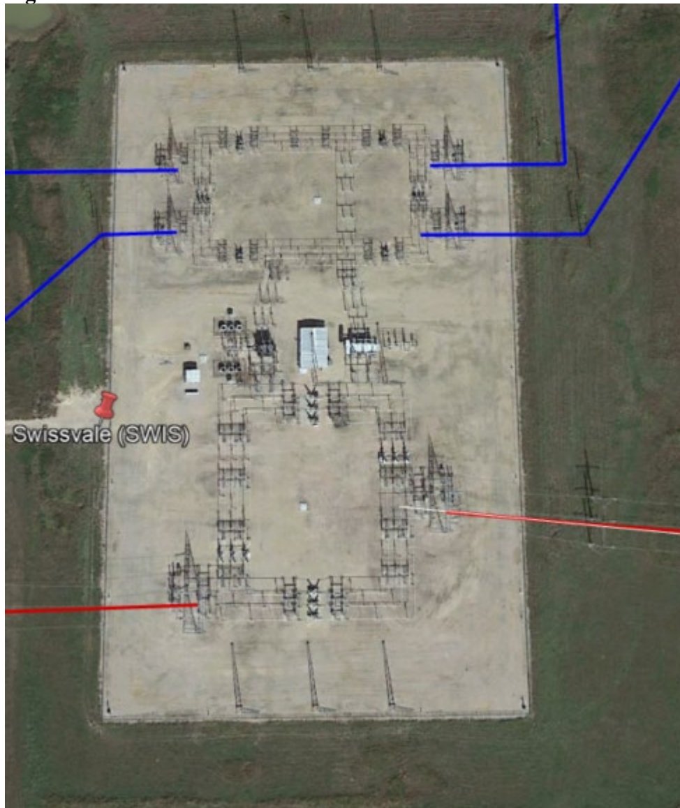
Figure 25 – Swissvale 345kV Substation
