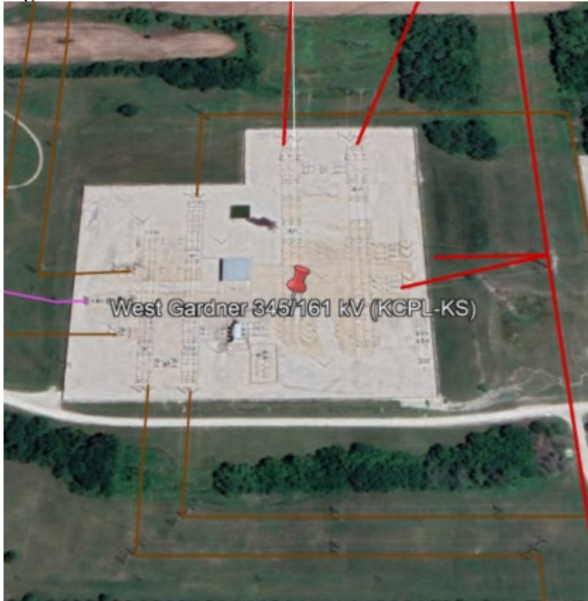
Figure 24 – West Gardner 345kV substation
